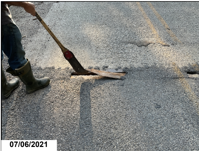
Metal plate at joint needs cut out and repaired At beginning of bridge
