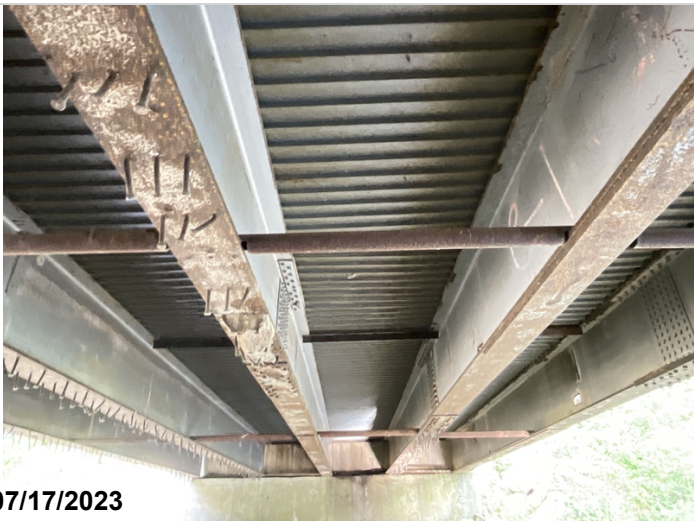
Underside of deck with stay in place forms
