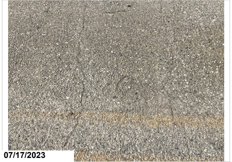
Deck cracking
