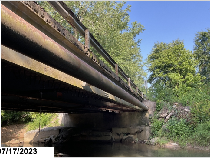
Utility pipe attached to steel beams. LT side of bridge
