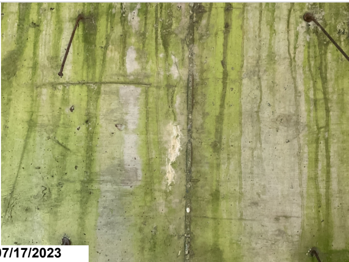
Cracking with efflorescence
