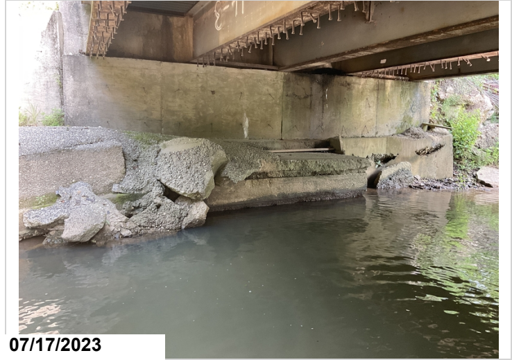
Bent 1 isolated scour
