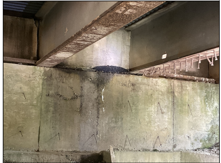
Asphalt on abutment 1 cap
