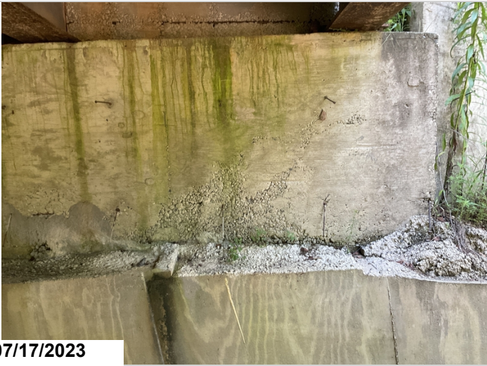
Abrasion on abutment 2
