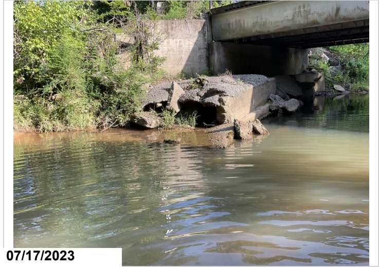
Bent 1 isolated scour
