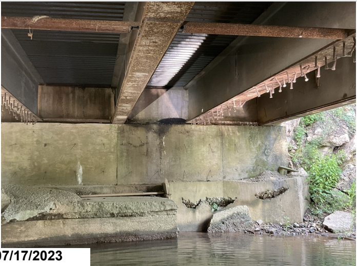
Asphalt on abutment 1 cap
