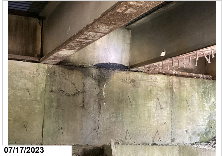
Asphalt on abutment 1 cap
