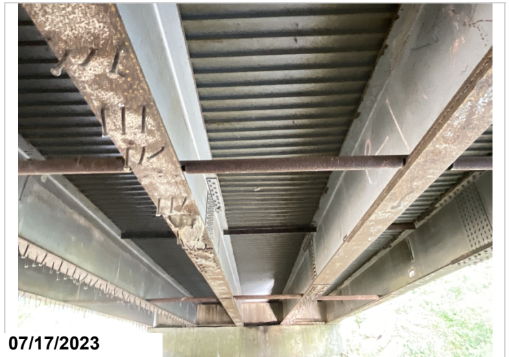
Underside of deck with stay in place forms
