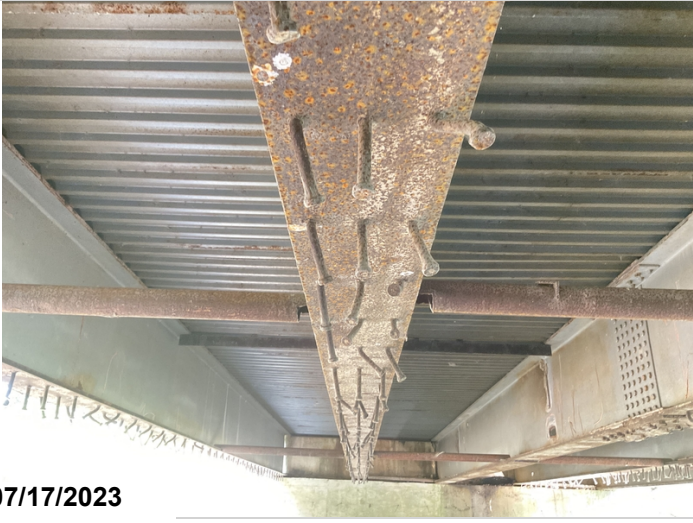
Corrosion to beams.
