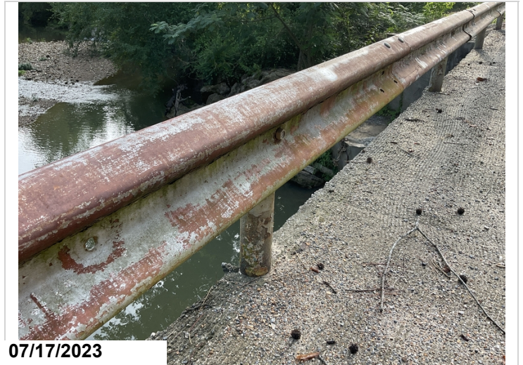
Corrosion on guardrail
