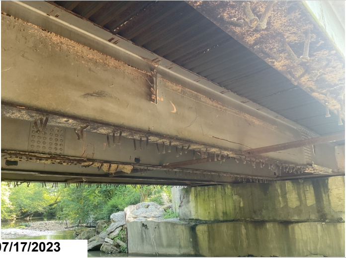
Shear studs on bottom of beams
