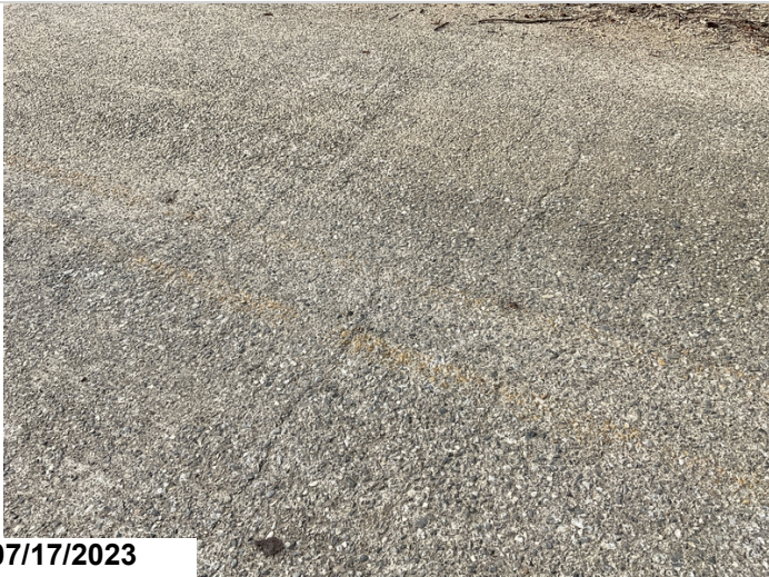
Deck cracking
