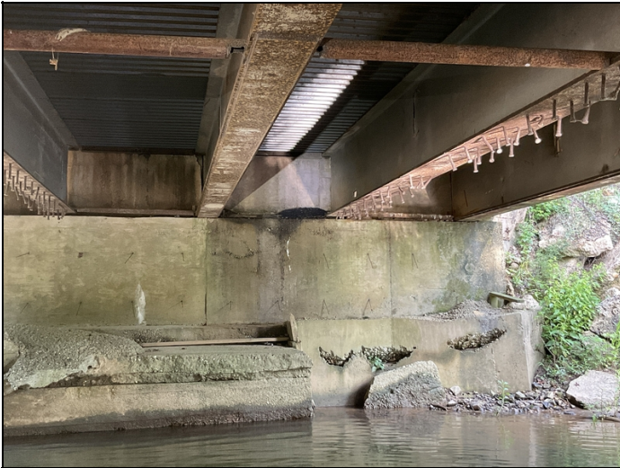
Asphalt on abutment 1 cap
